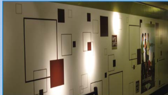
Wall Mural Installation
